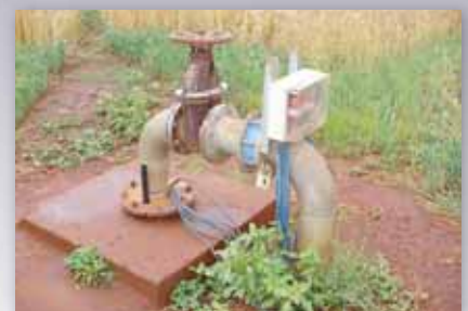
The completed installation of a borehole outlet pipe being fitted with earthing and surge protection units housed in the junction box. Note the sealed weather-proof junction box.
