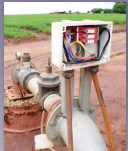
A closer view of the wiring and surge protection products in the junction box.
